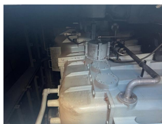
Turbine package, combustor / casing detail
