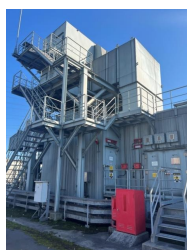
Package exterior, auxiliary modules and platforms
