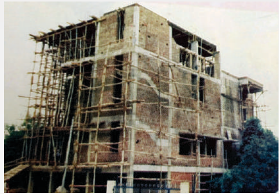
Church Construction in Progress
