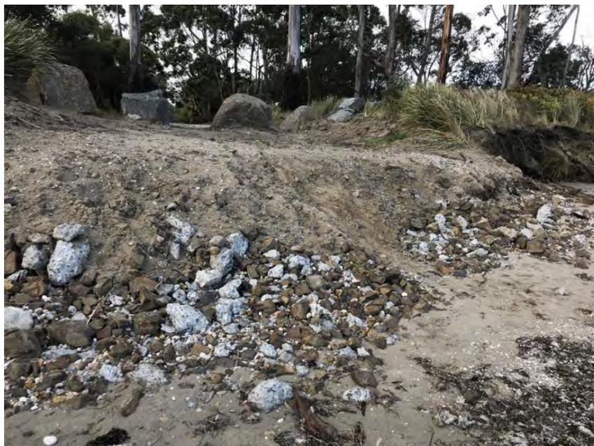
Figure 4. Drop off left after the removal of the boat ramp in 2019.
