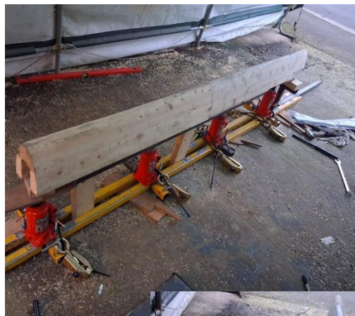
Stretch frame all welded and ready to go. Jacks fitted. Just to fit the anchor bolts and blocks, and away we go.
