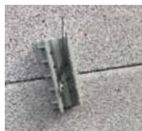
fixation using thin wire binding
