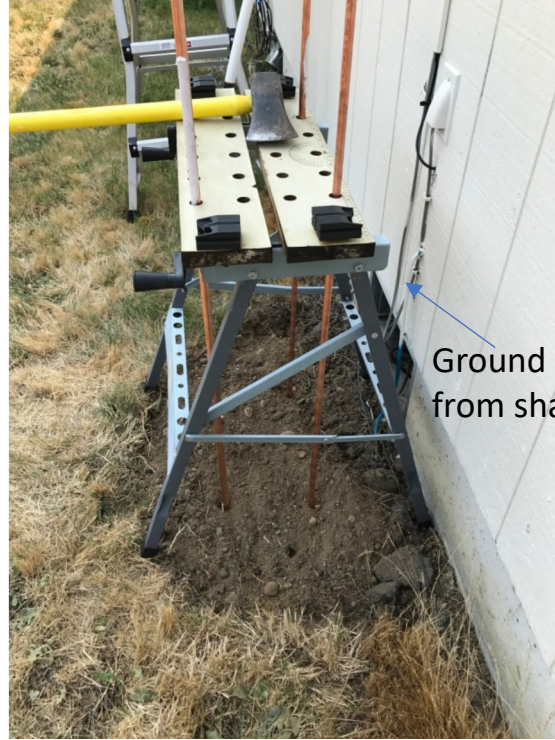
Sawhorse to hold and align ground rods
