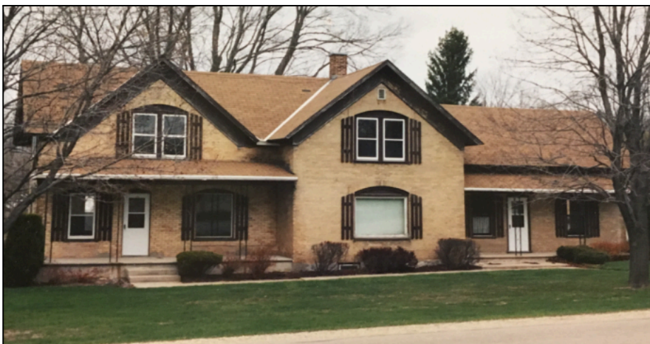
Parsonage after additions and renovations. Located to the west of the present-day church.
