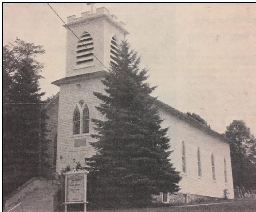
St. Paul Lutheran Church, Town of Washington after 1935 with the steeple removed.
