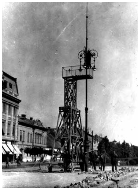
Installing pillar for street lighting in front of the city hall
