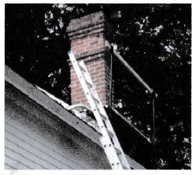
Chimney at the Historic First Baptist Church in Minnesota City.
