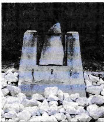
Rip rapping around the Swinging Bridge Pier (Oaks side)
