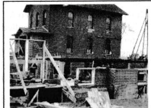
Photo of the 1938 Building under construction.
