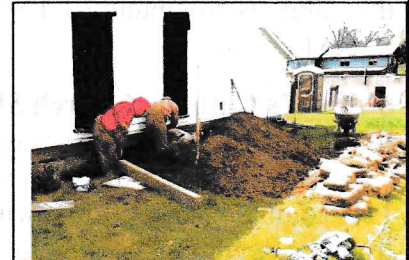
Jurowski Co. employees work on First Baptist Church
