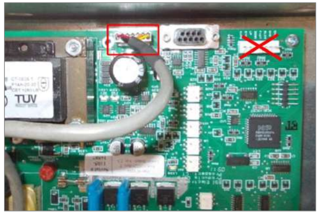
Fig. 46 Mercury/Path assembly, connection 4
