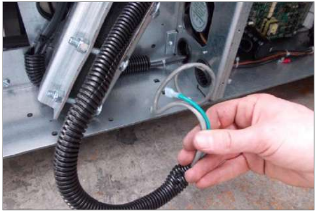
Fig. 43 Mercury/Path assembly, connection 1
