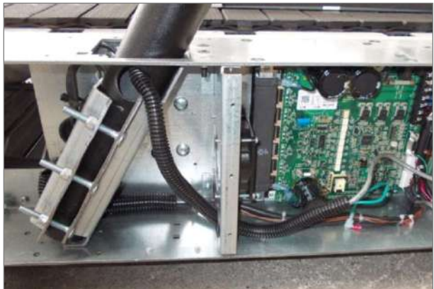
Fig. 44 Mercury/Path assembly, connection 2
