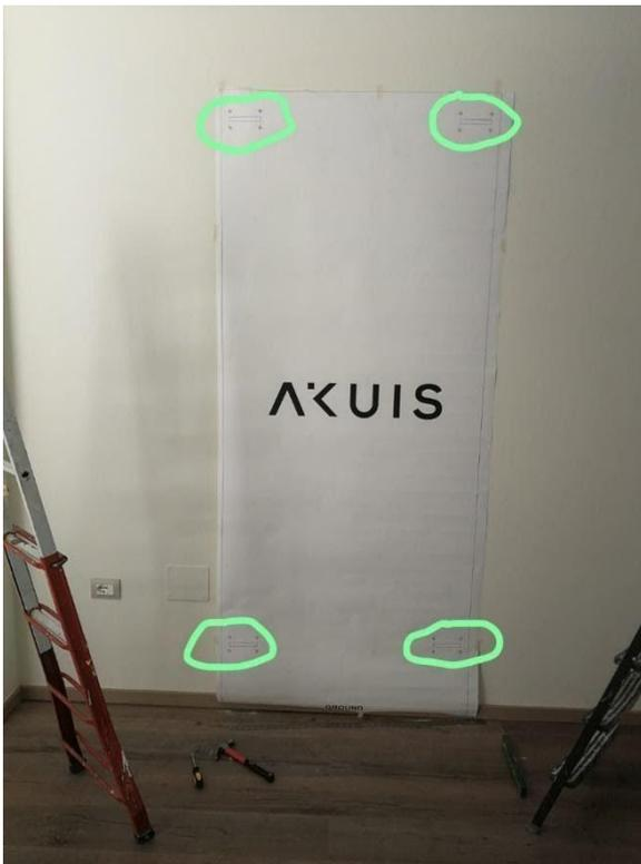
well with the horizontal line and smooth it out perfectly then fix it temporarily with sticky tape. The points where you need to drill the holes are highlighted in green in the picture. The bottom part of the template (under the word Ground) must almost touch the floor. This ensures optimal positioning of the equipment.
