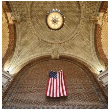
Guastavino tiled ceiling at the Yonkers train station.
