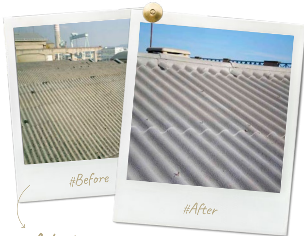
Asbestos Encapsulation
