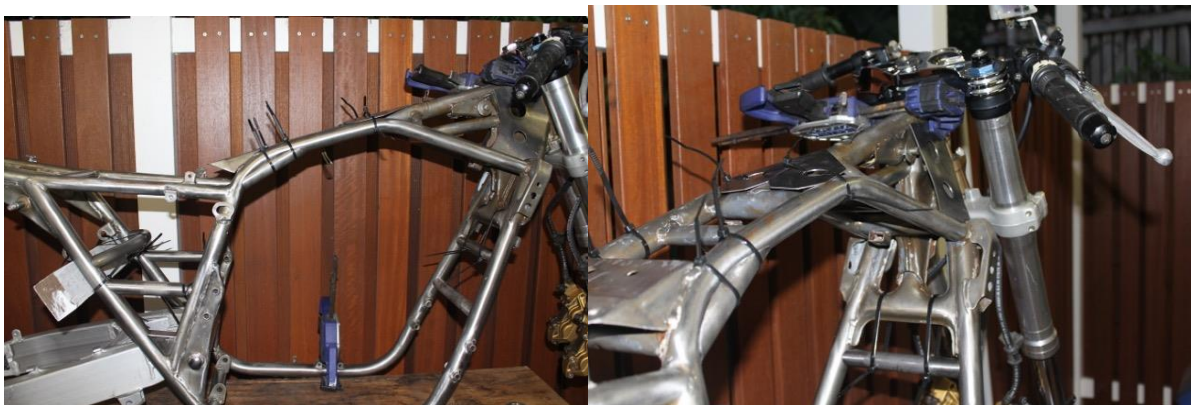
Photo #5 - Angles to be welded in main & down-tube
