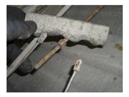
Let's clean the area where we will attach the plate well, using a wire brush, sandpaper, a chisel if there is rust... whatever it takes to make it hold on tight.
