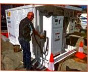
Whilst refueling, if excessive fumes and/or leaks are detected from pump or hoses, IMMEDIATELY hit the emergency button (as pictured), DISCONTINUE use and REPORT to office or supervisor.
