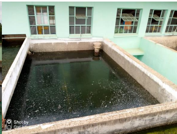
Flocculation tanks
