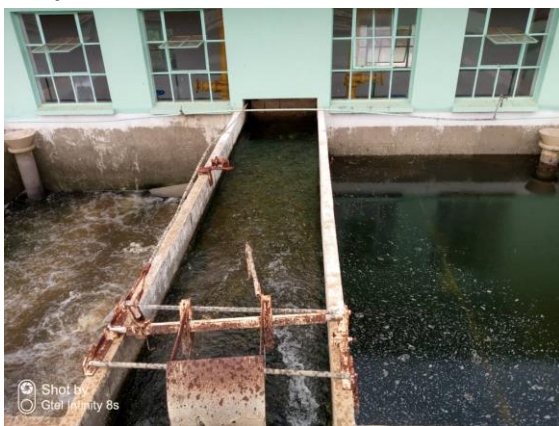
Alum Dosing Chamber
