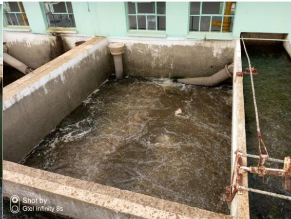
Flocculation tanks
